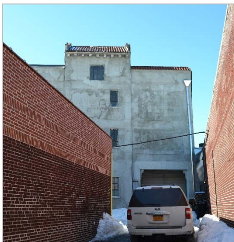
Existing building access alley looking west from Pondfield Road.
