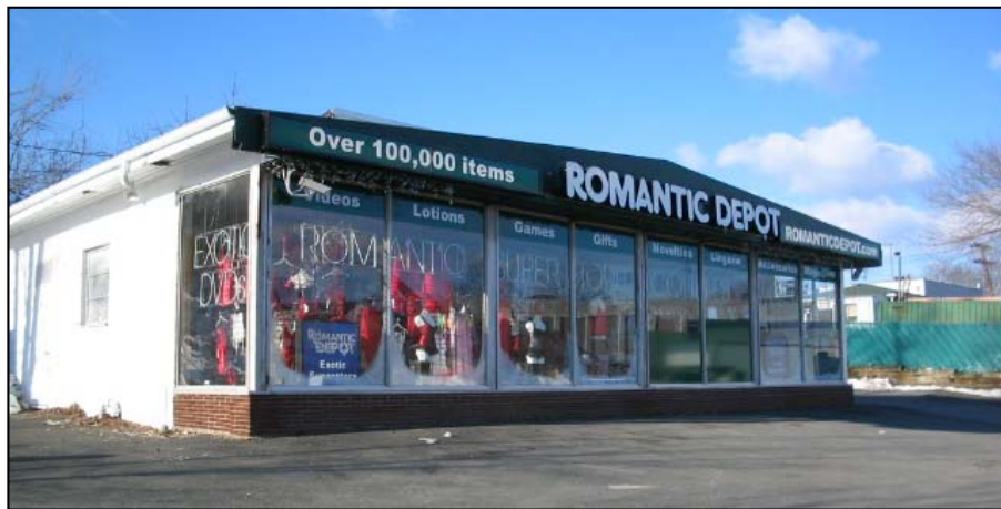
Existing Adult Use on I-287 Eastbound Ramp Elmsford, New York
