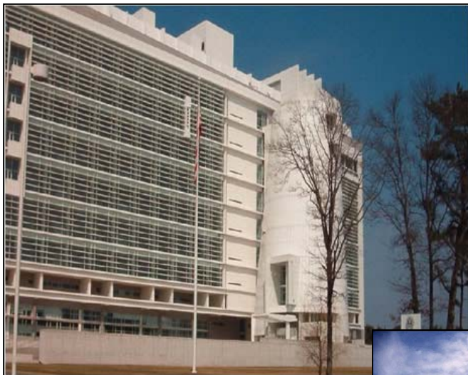
Alfonse D'Amato Federal Courthouse Central Islip, New York
