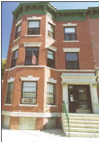
517 E. 187 th St., a renovated townhouse in Belmont.
