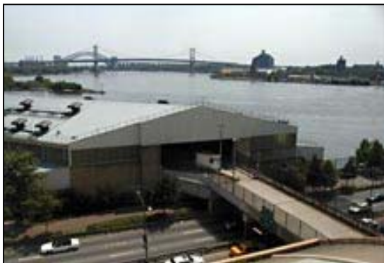
East 91st Street MTS as seen from the Upper East Side
