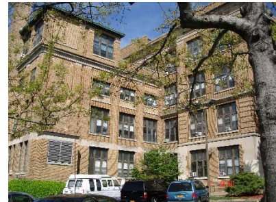
Washington House New Rochelle, NY
