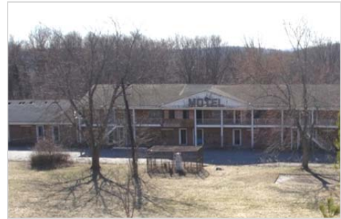
Abandoned motel on Project Site
