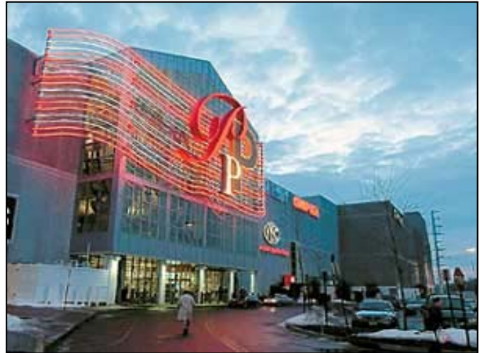
Palisades Center Mall, West Nyack, New York
